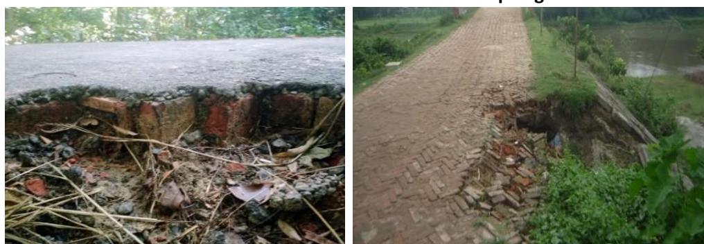
Picture 3: Road scheme without sustainable piling
